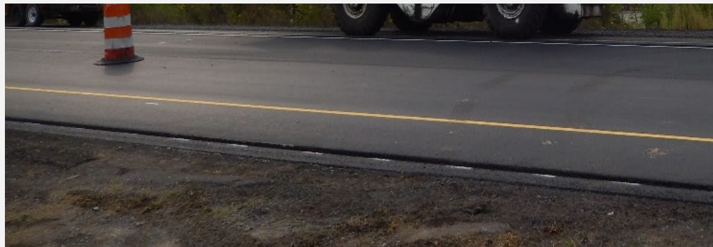
One-inch thick placed 6.3 mm, SR 220
